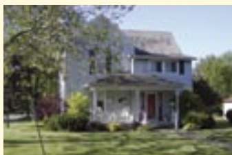
Moved from Harrison St. to 706 Van Buren St.
